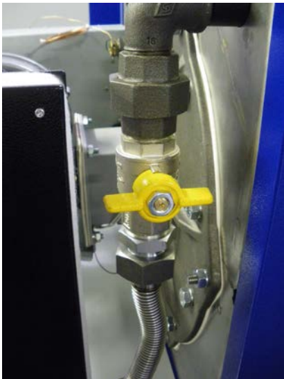
Figure 7.2.1 - Gas Isolating Valve (97 & 116 shown)
