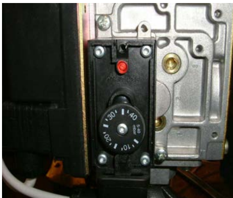
Figure 8.1.2 - Low Gas Inlet Pressure Switches
