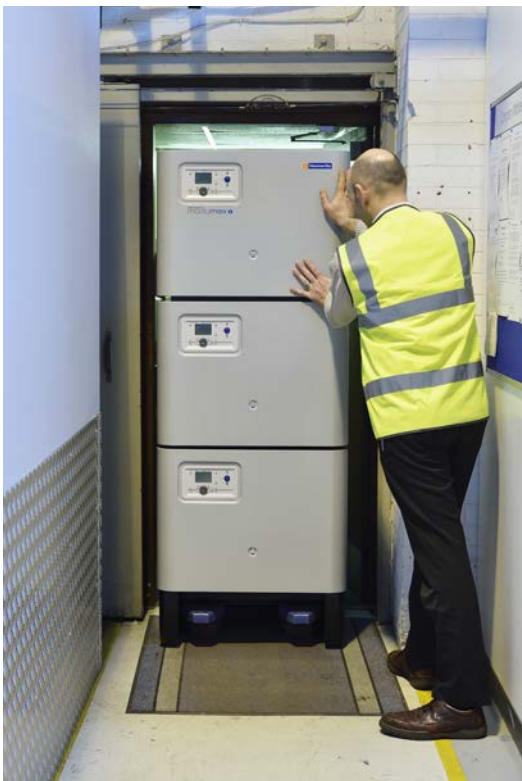
Figure 2.2 - Boiler Positioning
