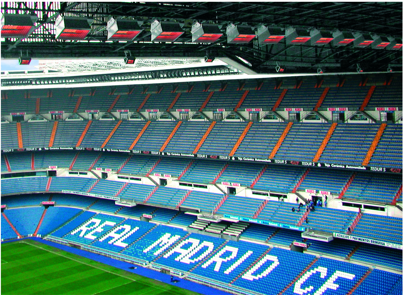
Real Madrid: 85,000 spectators capacity. Fully heated by 1,100 Schwank units. Highest mounting point at 55 meters.
