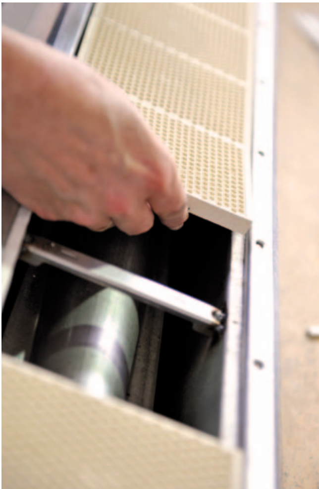
Lining of burners with ceramic tiles.
