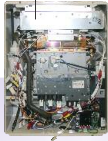
FASTflo – PLUS Condensing model Internal view
