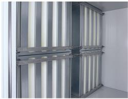
Air cleanliness is of particular importance in pharmaceutical applications. Air filters here fulfill a combination of several tasks: They protect staff and material from infections, and air handling units (AHUs) and the ductwork from contamination. Scrupulous checking of filters for clogging prevents the ingress of dust and cuts the operating cost of the system as the pressure drop across filters is reduced.
