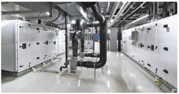
Air handling units by robatherm are especially designed to minimize the introduction, generation and retention of particulate and microbial contaminations in pharmaceutical cleanrooms.
